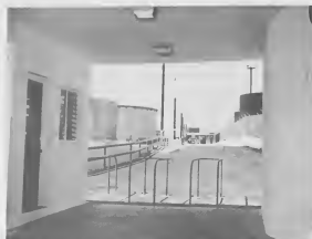
LAGO'S NEW refinery entrance will go into operation Tuesday morning, June 4. This photo was taken looking through the covered walkway to the Main Gate. Time card racks will be installed on the curved wall, right. Lago police will occupy the enclosure on the left; government police, the enclosure behind it.
